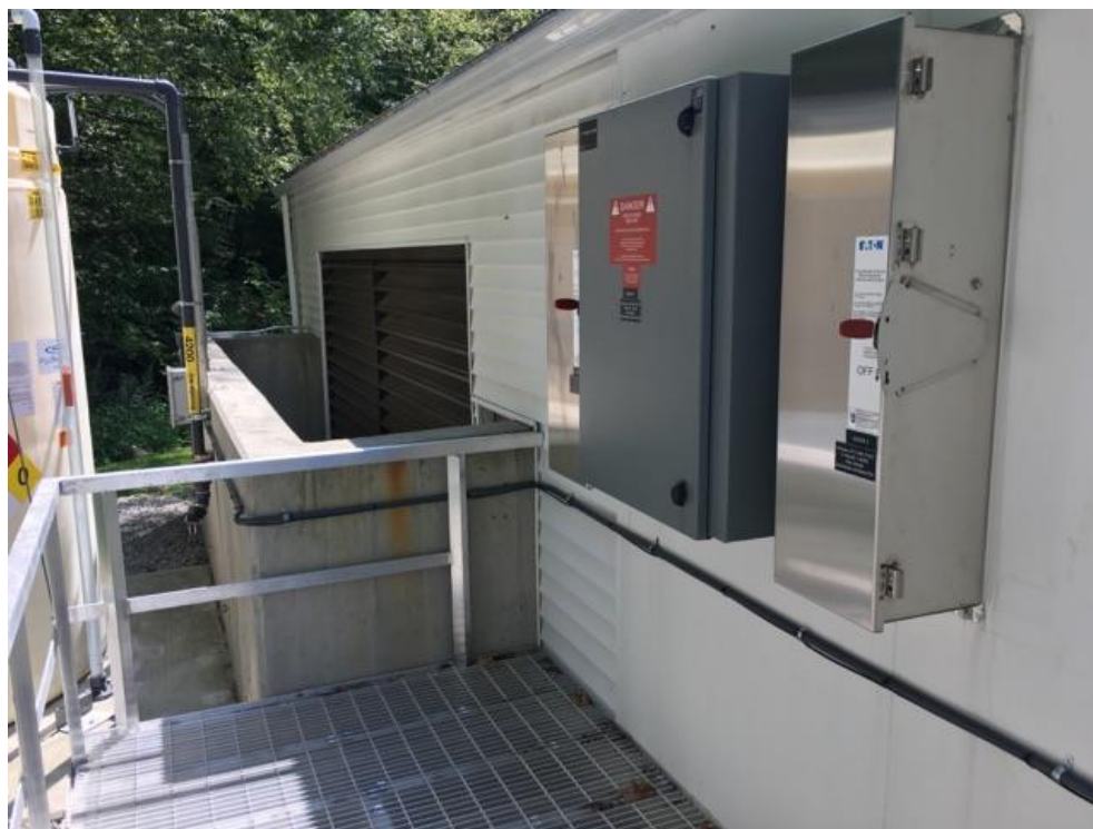
Figure 20 - Concrete Flood Wall and Raised Electrical Panels at Bolles Court Pump Station
