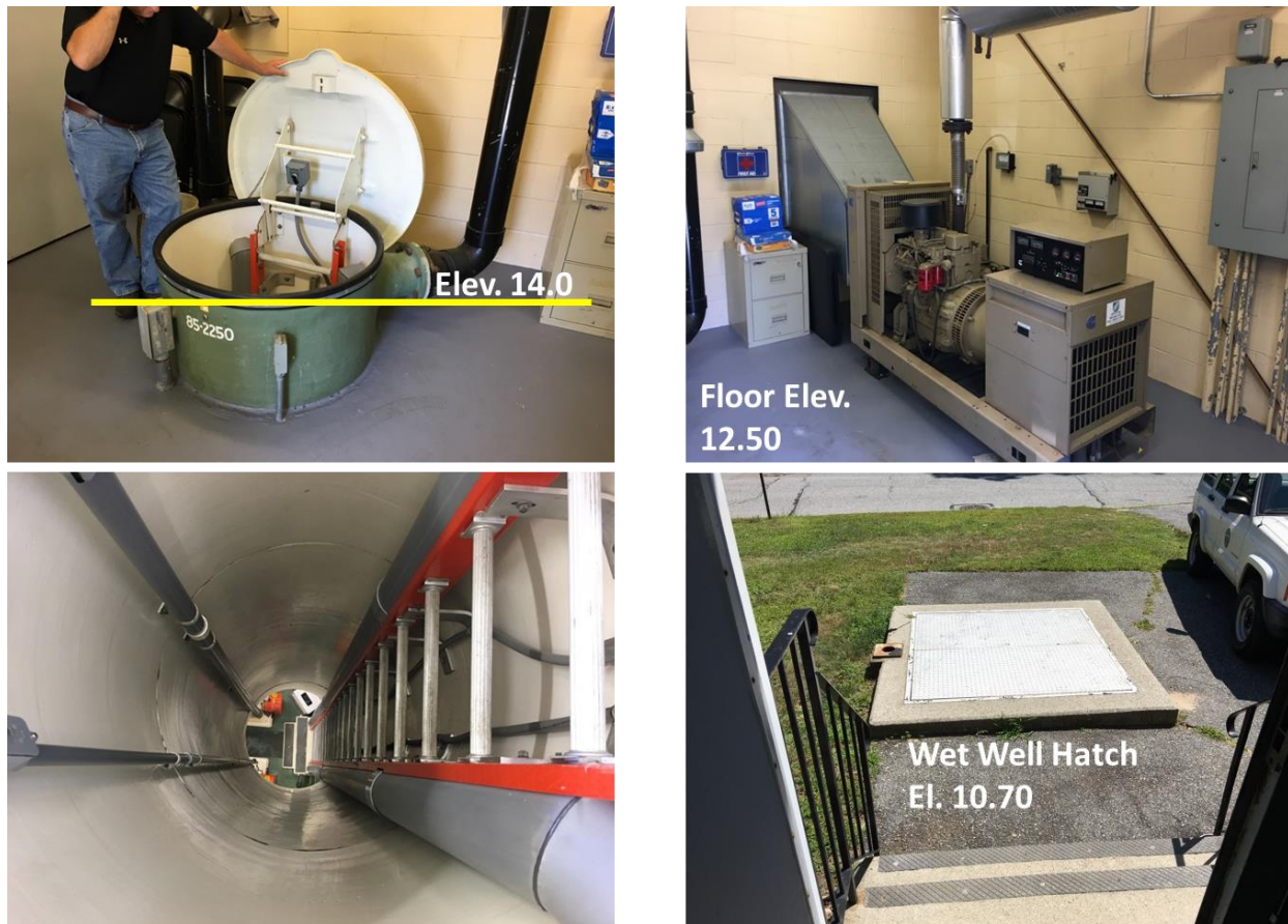
Figure 25 - Photos of Gardiners Wood Wastewater Pump Station
